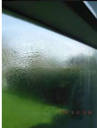
Figure 8 Active leaking/moisture, water stains, flaking paint, vapor seal breaks, etc. Recommend a window installer evaluate window for replacement/repairs and rule out any concealed damage.
