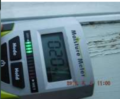
Figure 8 Active leaking/moisture, water stains, flaking paint, vapor seal breaks, etc. Recommend a window installer evaluate window for replacement/repairs and rule out any concealed damage.
