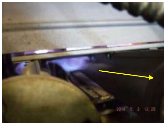
Figure 14 Example of flickering yellow flame and flame rollout when blower kicked on; have an HAVC contractor evaluate furnace for replacement (safety concerns).
